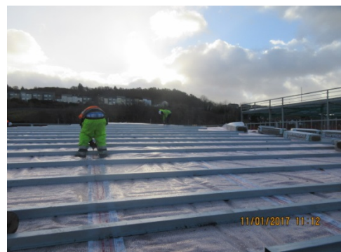
Photograph 4 Following completion of main structural steelwork the roof construction is ongoing
