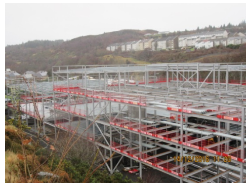
Photograph 2 – View of completed steelwork from rock outcrop
