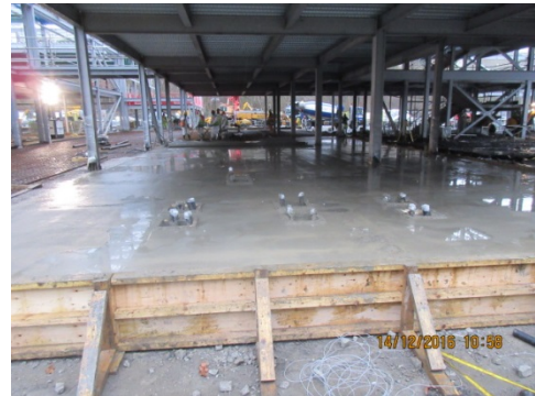
Photograph 8 Placement of concrete to ground floor
