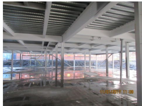
Photograph 10 Intumescent paint applied to internal steelwork
