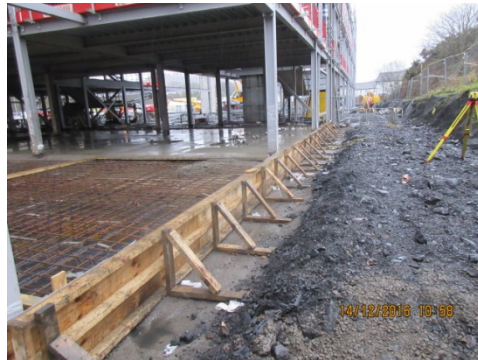
Photograph 7 Perimeter formwork erected for ground floor slab
